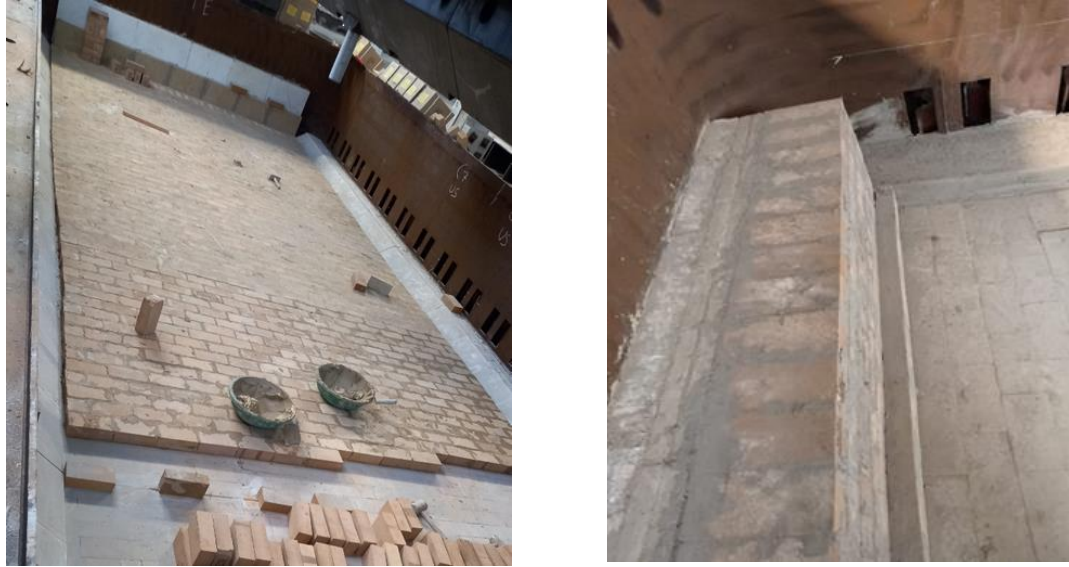
Figure 9. Lining construction. Left: bottom. Right: lower endwall.
