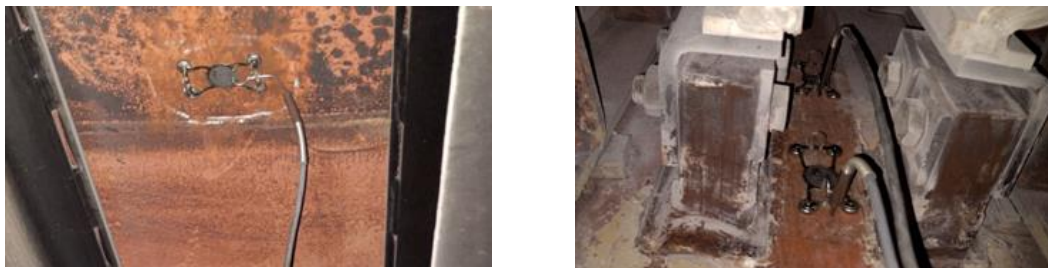
Figure 4. Heat flux measurements. Left: shell bottom. Right: shell between collector bars.
