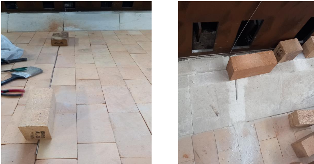
Figure 8. Thermocouple installation. Left: bottom. Right: lower sidewall slope insulation.
