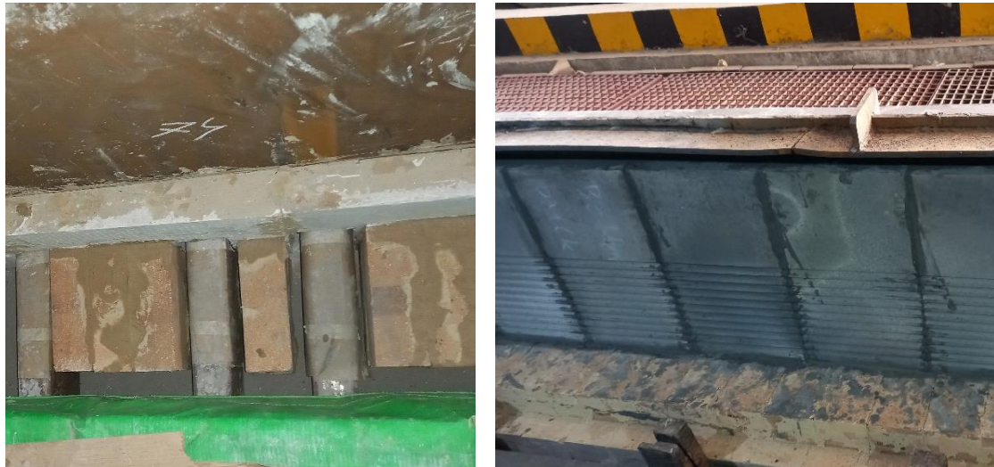
Figure 10. Lining construction. Left: lower sidewall. Right: upper sidewall.
